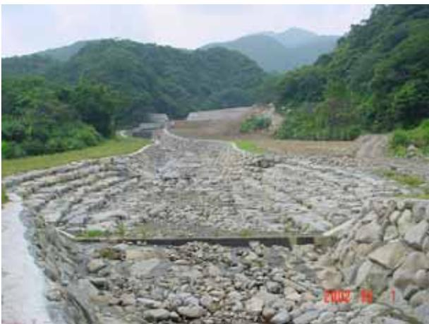
**Fig. 4 – Gentle slopes of streambank protection of Chung-ho Village in Taipei County.**
