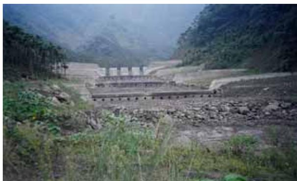
Fig. 15 – The No. 1 slit dam and series check dams.
