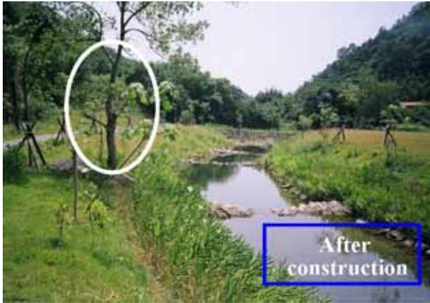
**Fig. 3 – After the flood during Typhoon Mindulle in 2004, the downstream of Shen-nong Bridge shows no damage and the river course becomes naturally meandering.**
