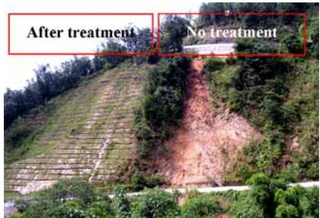
Fig. 13 – A comparison showing the effect of staking and wattling erosion source method.
